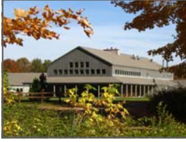
Dining Hall/Main Office
